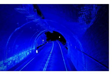
Using Hovermap, Brierley Associates was able to scan the tunnel at night, reducing safety-required closures and the impact to traffic while still capturing highly detailed data that can be used to inform remediation and rehabilitation recommendations.
