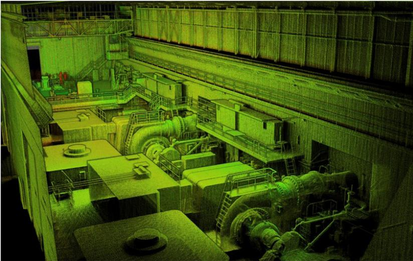
This pump house as-built was captured with a 5-minute indoor flight. Prior to the flight, the pilot demonstrated Hovermap's collision avoidance to assure the customer the drone could be safely flown around this critical piece of infrastructure.
